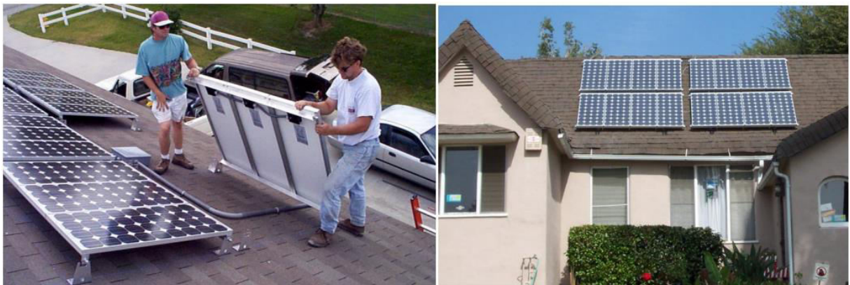
PV Installation on Roof
