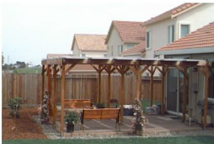
PV mounted on Patio Cover
