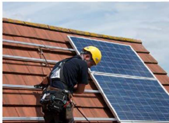
Sloped Roof PV Mounting Arrangement
